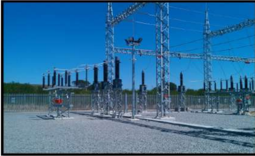
Construction of 132kV Substation
