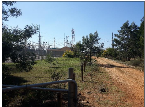
Photo 6: View towards east with entrance road to substation in foreground
