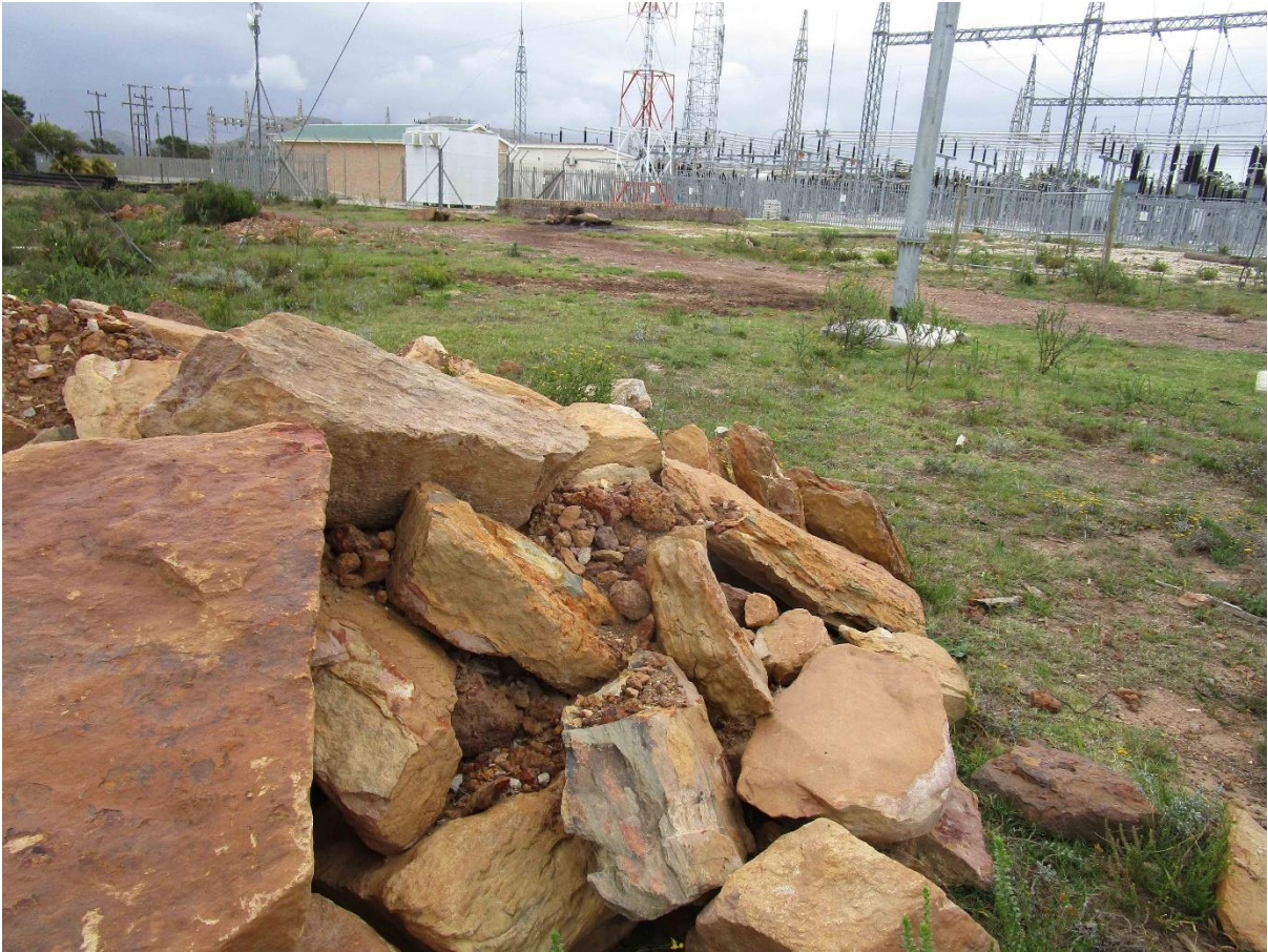
Figure 5: Piles of rock adjacent to the existing substation, excavated during its construction.
