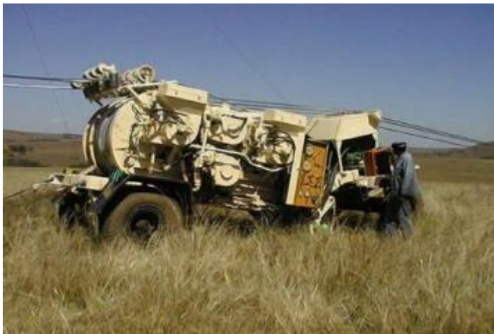
Figure 6: Mechanical stringing of conductors
