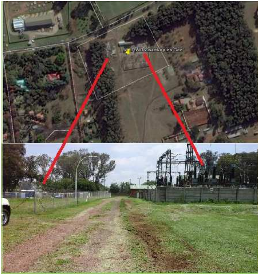
Photograph showing the proposed site for the expansion of the Zwartkopies substation
