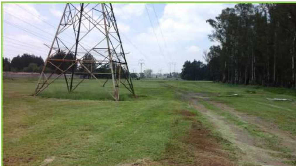
Photograph showing the existing 2x88Kv lines from the RWB Zwartkopies substation, also where the new distribution power line of 2.6km long with 22m servitude will be constructed.
