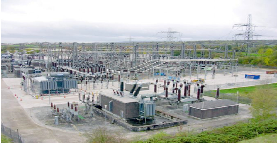
Figure 3:3 GIS is an open and thus cooled by the surrounding air
