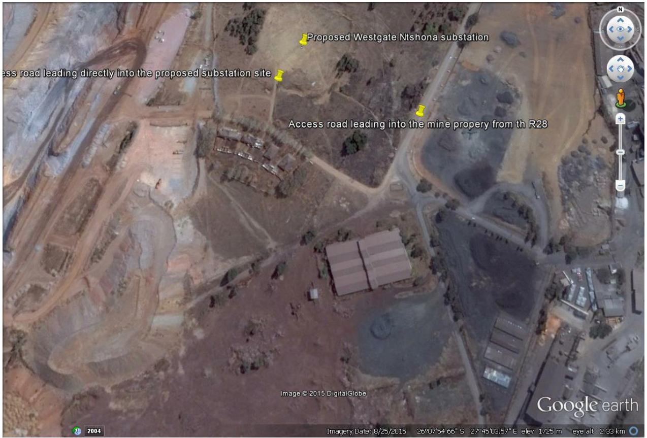
Figure 4: The existing access and dirt roads near and leading to the proposed substation
