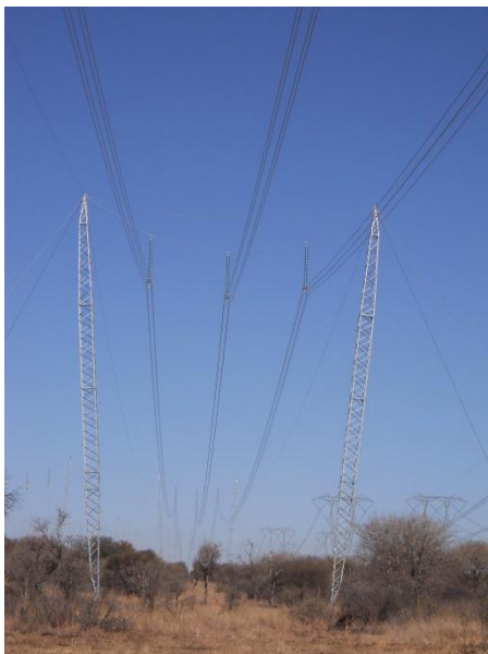
Cross-rope suspension tower
